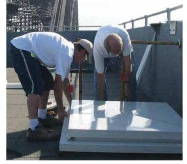
An all-metal Skyhatch is being installed at the south east pylon on the iconic Sydney Harbour  $\mbox{Bridge}.$
