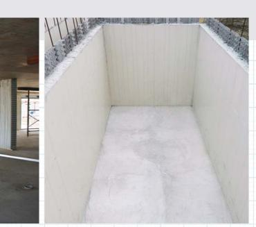
3 Step Installation Purpose-built braces are available for hire A single core fill is all that's needed for panels up to 3.5m
