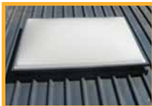
Metal Deck Roof Type
