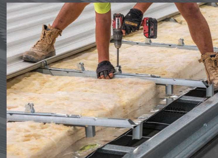
^ NO NEED TO SHORTEN THE SPACER TO FINISH THE ROOF
