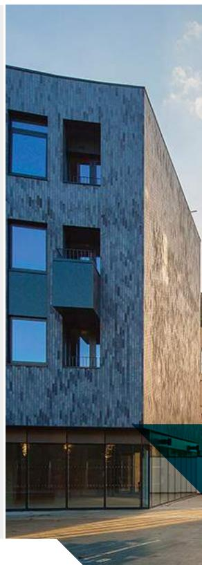
CORIUM brick tiles can be mounted at any angle to achieve truly dynamic finishes – even overhead for soffits and ceilings.
