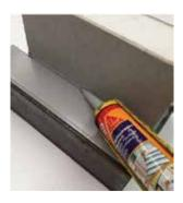
**4.** Apply bead of Sika between the edge of the UB flange and the UB infill.
