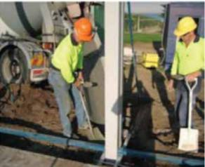
For long-life designs (\*\*\*) 25 years), a zinc-rich industrial preventative coating must be applied to the base of the footing and 100mm min. up the base of the post. MWS recommends "Dulux Durebild STE", applied thickly (100µm min.).
