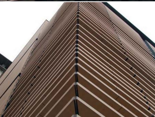
UCL London, GB Architects: Grimshaw and Partners, GB Façade system: MOEDING ALPHATON® Colour: beige patinated Special shape: baguettes
