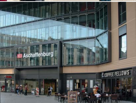
Aschaffenburg central rail station, Aschaffenburg, Germany Architects: Architekturbüro Kammerl + Kollegen, Pfaffing Façade system: MOEDING LONGOTON® Colour: special colour Special shape: baguettes Surface: standard, grooved
