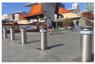
Vehicle access to the site is controlled by two sets of LEDA stainless steel *automatic retractable bollards* which can be controlled and accessed through intercom or card. In this instance our WA office and client chose electro mechanical operated bollards.
