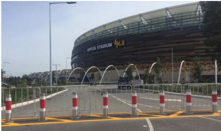
The bollards normally remain retracted and are able to be raised limiting vehicular access during events. Choosing semi automatic retractable bollards over fully automated systems saved many hundreds of thousands of dollars on the project.
