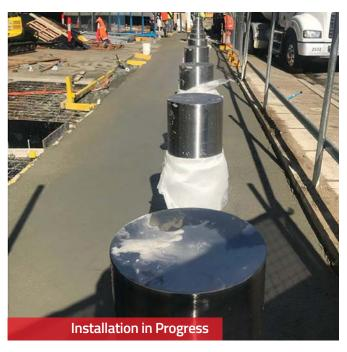
This problem is solved with LEDA's *shallow mount bollard* systems. Requiring only a 114mm deep penetration, LEDA's bollards provide the shallowest footing available in Australia, while still providing a PAS68 rating for a 7.5Tonne vehicle at 80 km/hr.
