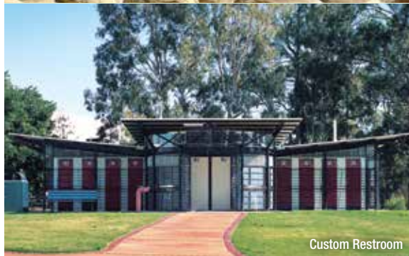
Modified K9500 Caretaker Restroom
