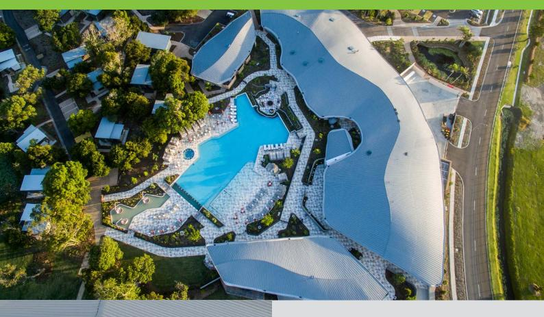
Each sheet was individually rolled and shaped so that all seams pointed to two control points on either side of the pool.
