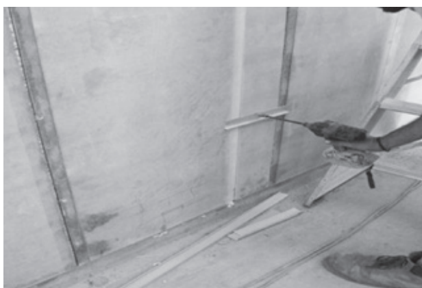
Fix a toggle (ply wood or aluminium angle) to the tee junction bringing it flush with adjacent panels.
