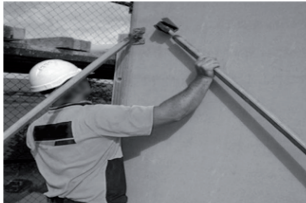
Secure brace foot plate to slab with Excalibur bolt and brace to panel with self-tapping screws into panel stud. Proceed to plumb panel in all directions utilising the brace's push pull mechanisms and a level.
