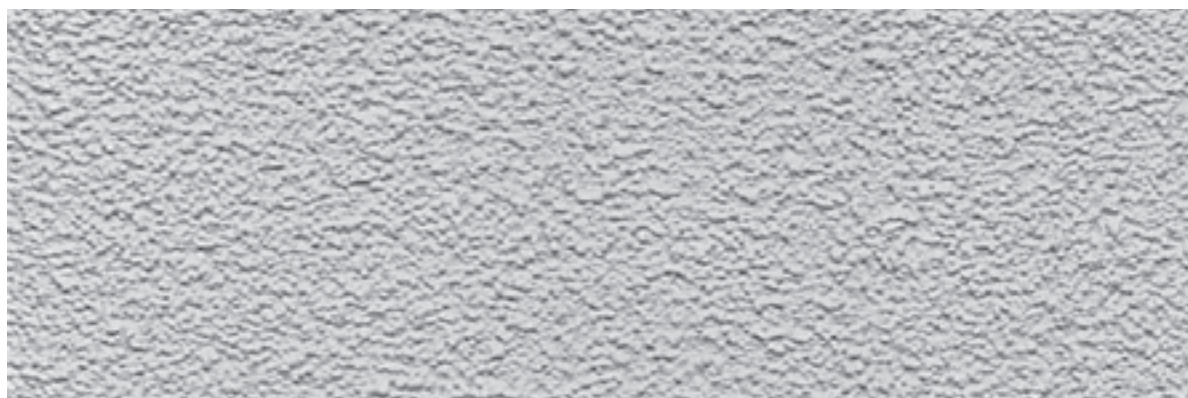
TYPICAL TEXTURE COATING FINISH
