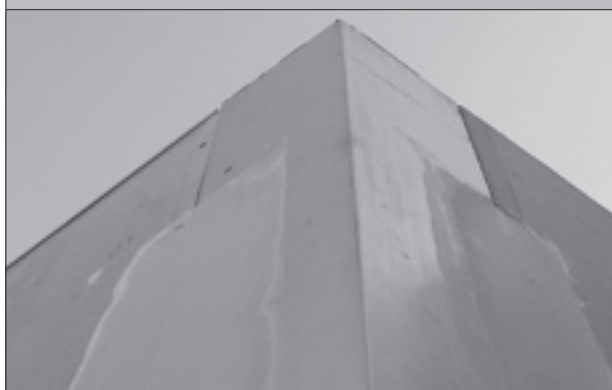
BASE COAT APPLIED TO CORNER CLOSER FIGURE 5.7
