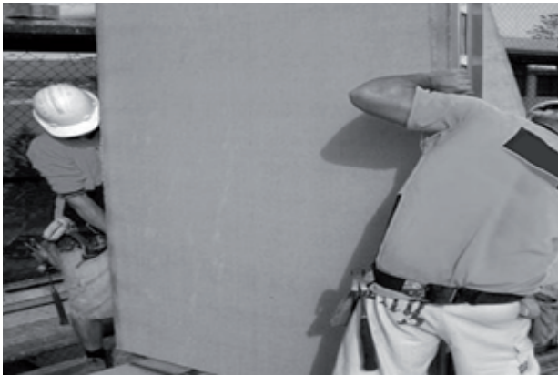
Position first panel in line with surveyor's wall starting point.
