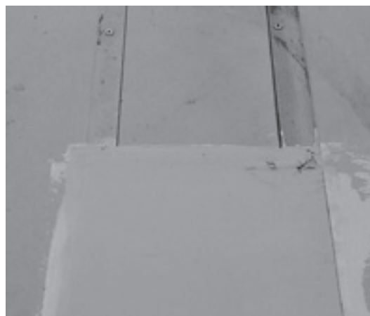
SETTING OF T-JUNCTION CLOSERS FIGURE 5.10
