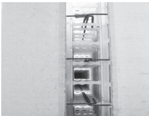
Ensure panels are plumb in all directions and screw off internal corners. Ensure that all horizontal and vertical reinforcement has been fixed to engineers specifications.
