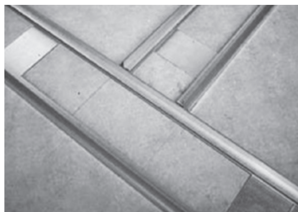
T-Junction Bottom Plate Set-out
