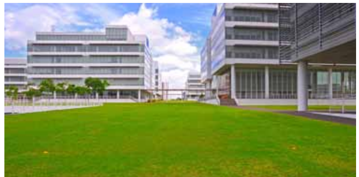
Fire Engine Access
