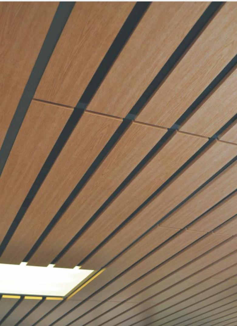
**Grid Requirements:** Existing grid may be repainted (enamel paint recommended) and used but must be able to support the weight of the tiles as well as the service load factors as prescribed in the AS2785. Refer to Supawood's Technical Services Department for tile weights.
