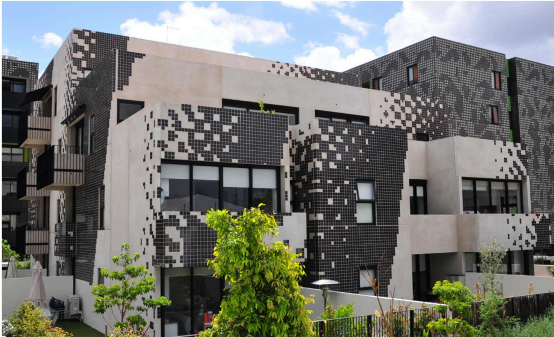
Our thin brick inlay system involves laying thin bricks or stone of varying sizes into precast concrete to quickly achieve the look and feel of a traditional brick, stone or texturised wall. Plus you enjoy all the efficiencies of precast concrete – reduced cost and installation time, easier site management and an innovative, contemporary wall solution.
