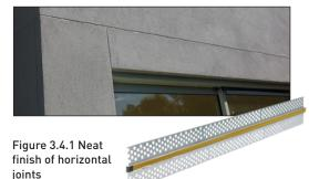
The external aluminium render bead can be used as an option at horizontal joints to provide neat and consistent finish joints. After installation of the PowerPanel<sup>XL</sup> panels, the render bead is applied and hold onto place by using Hebel adhesive. Suitable external grade sealant is to be applied at the joint before rendering.
