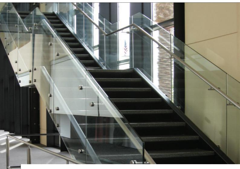
CRL is now manufacturing Standoff Railing Systems. By specialising in the design and manufacturing of this innovative system, we offer you the ability to create custom railings that will address project-specific criteria. Rest assured that the products we offer will represent the current evolution of the railing industry because product development is an ongoing process at CRL.
