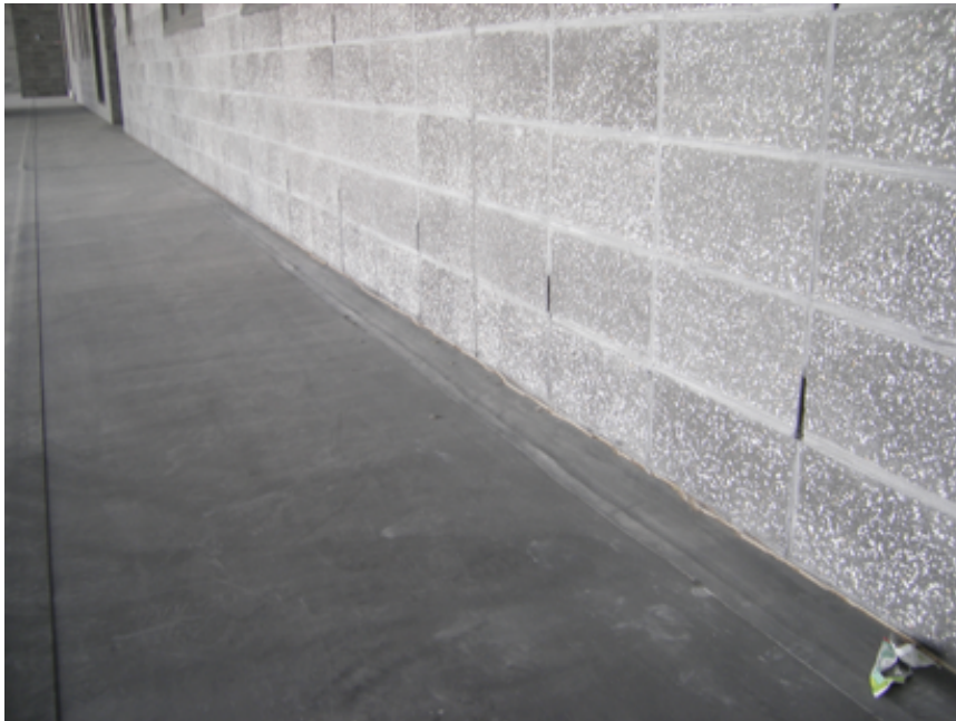
The Wolfin membrane system continues under the block façade to form the cavity flashing
