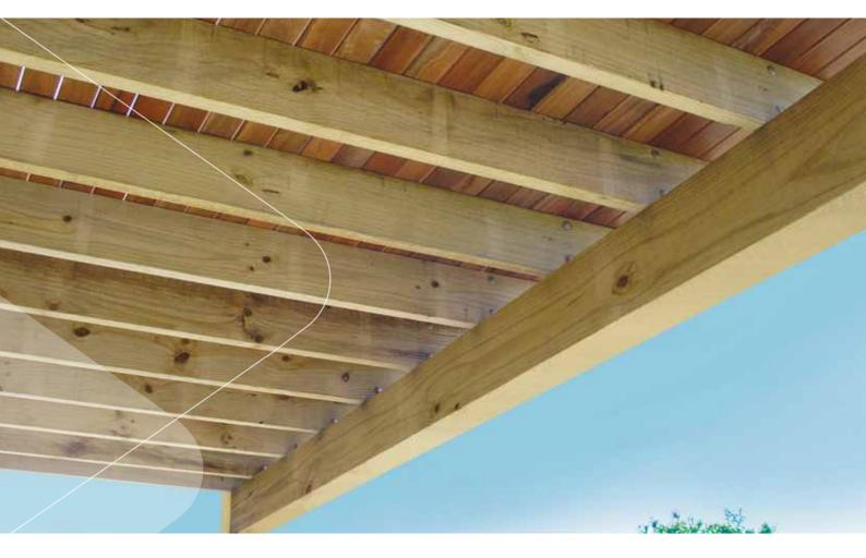
The selected MGP10 grade and unique H3 treatment makes Hyne T3 Green the new generation structural timber for external, above ground use. Offering a combination of guaranteed strength, improved stability, consistent reliability and outdoor durability, Hyne T3 Green provides real value for builders, architects, designers and for timber merchants who stock and supply outdoor timber.
