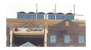
Skyspan Barrel Vaults can be glazed in a range of acrylic or polycarbonate tinted sheet materials. Opal, clear, bronze and grey solar tints provide the main range of hues. The use of fabric sails enhances the aesthetics and provides regular shading.
