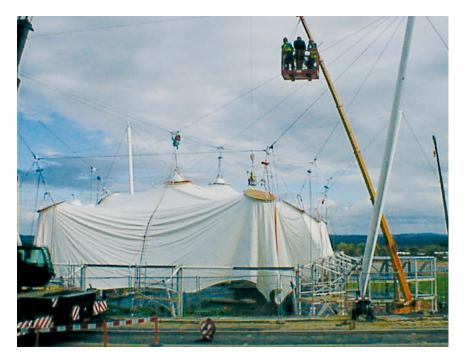
Installation phase for a high point shaped membrane roof. This process requires to be integrated into planning phase and must be carefully synchronized in the whole installation concept. Therefore only in tensile structures it is possible to cover 2000m<sup>2</sup> surface within 5 full days installation time.
