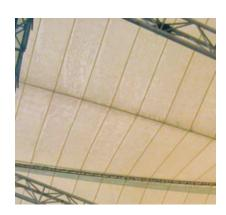
Image 2: Lacquer adhesion problems in translucency. Where lacquer is not performing the coating is directly exposed to soiling and UV attack.
