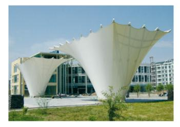
Example of asymmetrical curvature shapes with symmetrical primary structure, only generable by using VARIO-STRETCH fabric, properly compensated.
