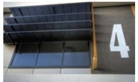
While the standard grating is manufactured using a 45mm x 3mm extruded aluminium blade, due to its simplicity of design it can be manufactured differently to suit a project.
