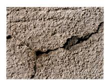
Weathered and deteriorated masonry structures have long represented one of the most difficult maintenance challenges for the contractor. In the past five years, recoating with an elastomeric wall coating has become one method for repairing these surfaces.
