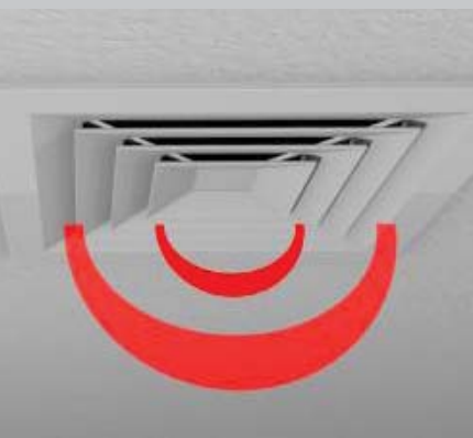
Unwanted sound easily travels through any perforation such as lighting or ducting.
