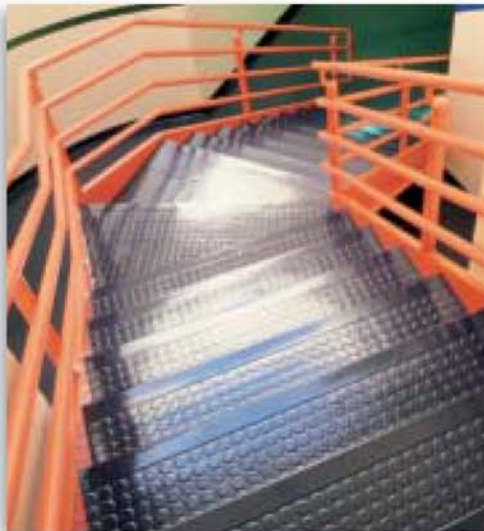
Vista Detention Center, Vista, California
