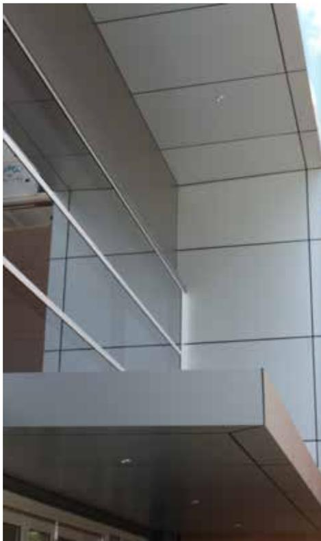
AODELI HCP is oriented from the Aviation industry. It's durable, large span and super flat. HCP also features in fabrication-friendly, multiple surface solutions and colour options. It is widely applied for Architectural area such as façade, roof, partition as well as transportation, voyage and equipment industry.
