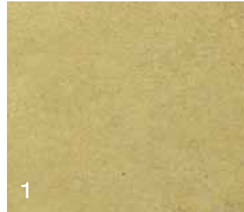
Machine trowel finish
