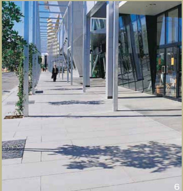
6 Charcoal coloured concrete was laid and then subsequently saw cut to create an extremely durable and interesting pavement along this inner city tourist facility. CCS Black 21 at a 4% dose rate was specified.
