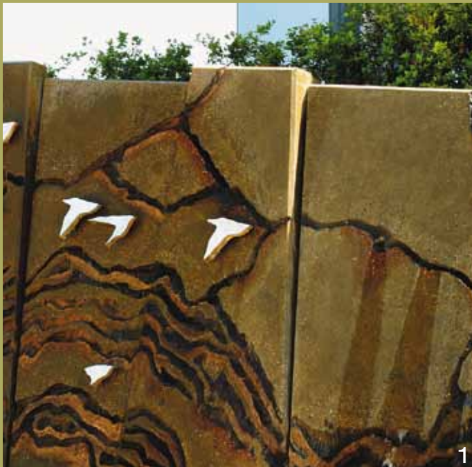
1 This uniquely designed wall was created with the use of CCS Bonsai (together with a reactive stain) and distinctively formed shapes made from polystyrene. Landscape Architect: Urban Art Projects.
