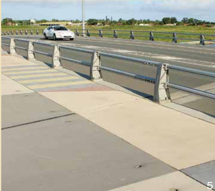
5 Adding colour can liven up an otherwise plain concrete bridge. Colours: CCS Driftwood, CCS Nougat and CCS Onyx 21 in conjunction with red and yellow coloured pavers. Landscape Architect: Gamble McKinnon Green.
