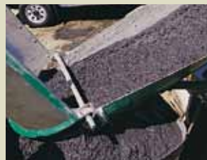
3 After sufficient mixing, coloured concrete is discharged from the concrete truck.
