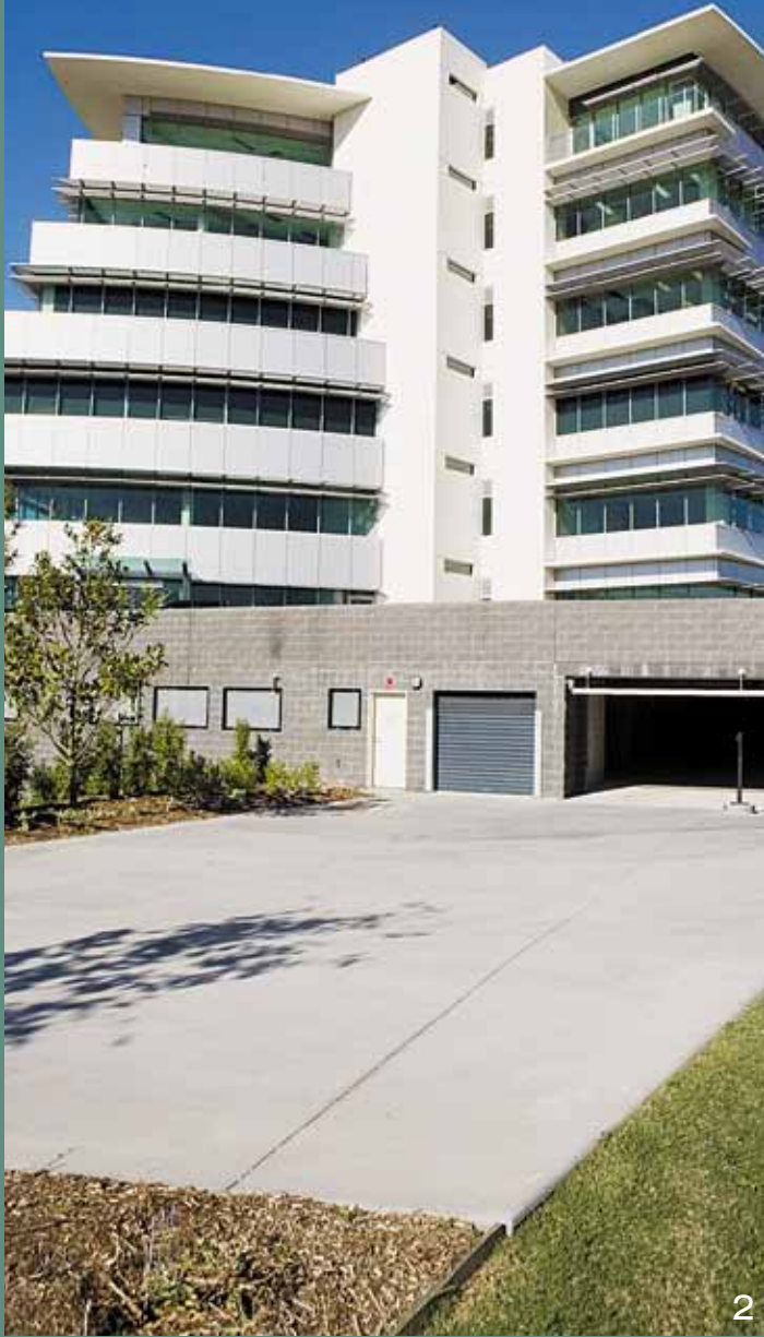
2 This energy efficient building facade was created using CCS Snow pigment in off-white cement to provide a permanent, low maintenance finish. CCS Black 21 was used to provide a low glare, functional path and driveway. Architect: Atelier Group Qld.
