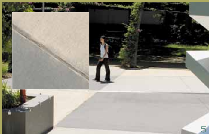
3 Coloured concrete was laid in a staged manner to create contrasting colours in a small area. CCS Corn, CCS Pewter and CCS Bluestone. Project: James Street, New Farm. Architect: Cottee Parker Architects, Brisbane.
