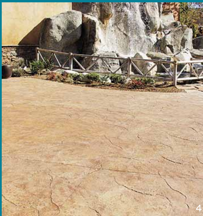
4 This weathered stone look was achieved with the seamless CCS Sierra stone mega mat.
