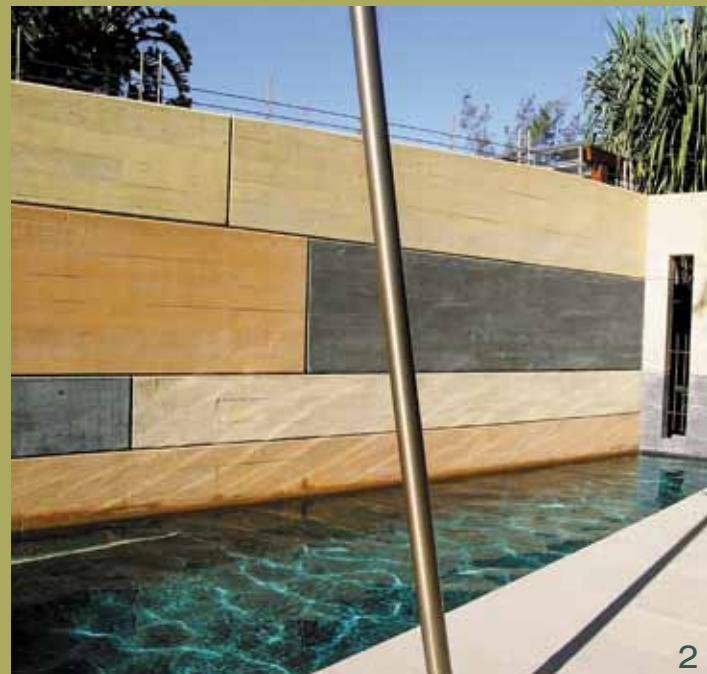
2 Panels coloured with CCS Lemon Cream, CCS Tangerine (special blend) and CCS Black 21 combine to provide a bright, contemporary off-form wall. Architect: John Mainwaring (JMA).
