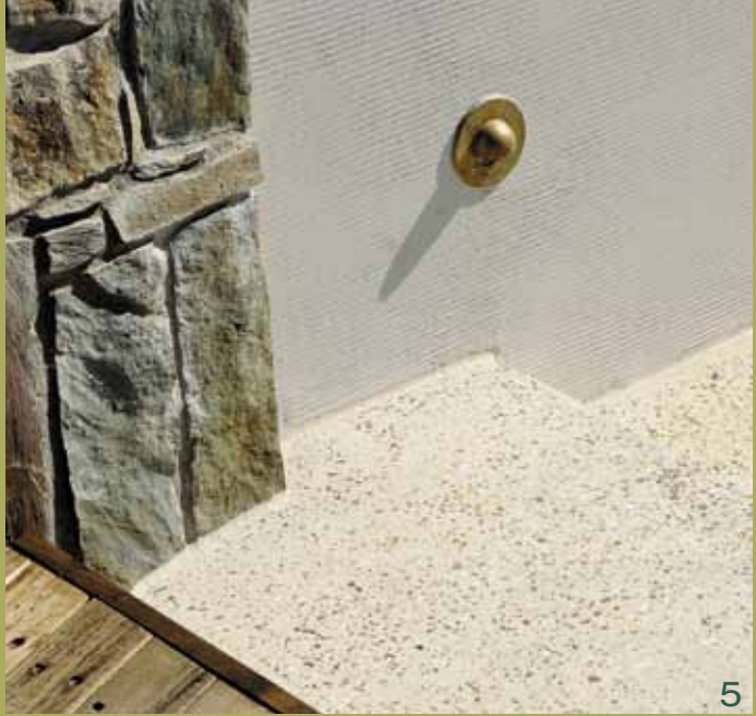
5 A lightly exposed concrete finish (coloured with CCS Parchment) is a functional and attractive look for these steps at Ephraim Island Resort, Qld. Architect: Edaw Australia.
