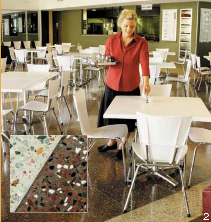
2 Special blends of CCS pigments were combined with natural stone, in this concrete blend. Both were revealed to their full beauty when the concrete surface was subsequently polished and then sealed.
