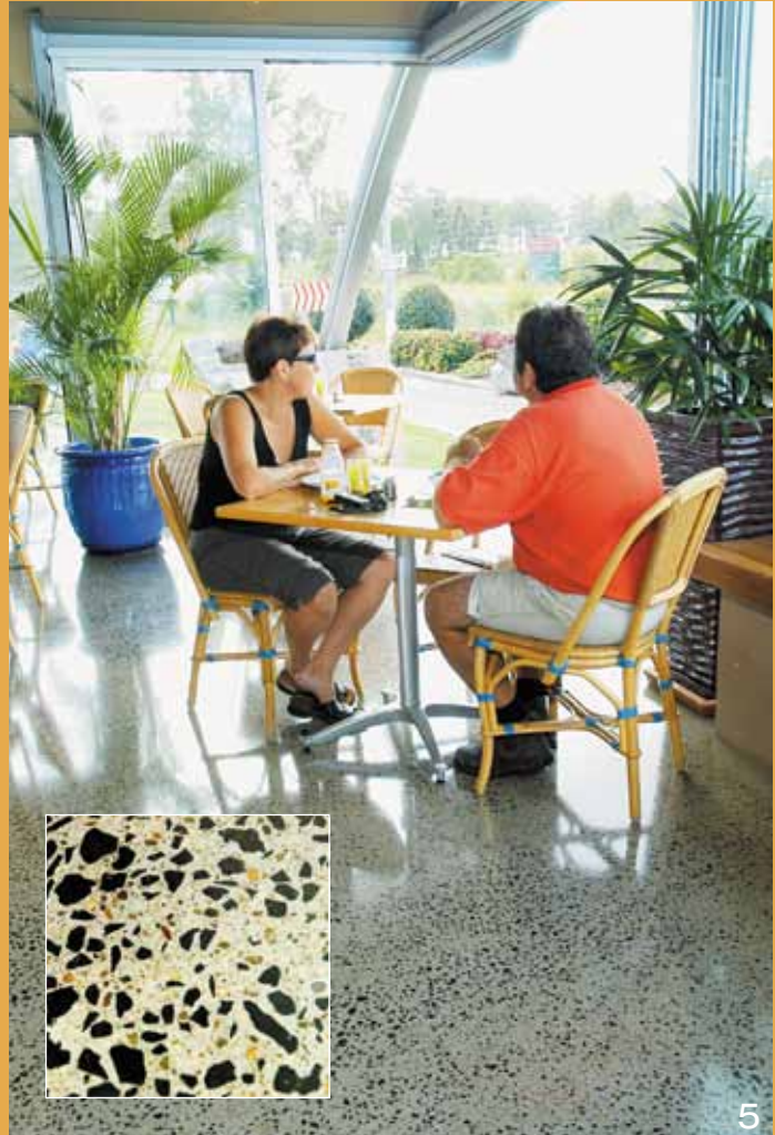
6 The Direct Factory Outlet Centre in Brisbane incorporated polished concrete within the main thoroughfare areas. A distinctive but similar coloured aggregate to CCS Lemon Cream was used to provide the contrast. Architect: S.P.L.A.T. Qld.
