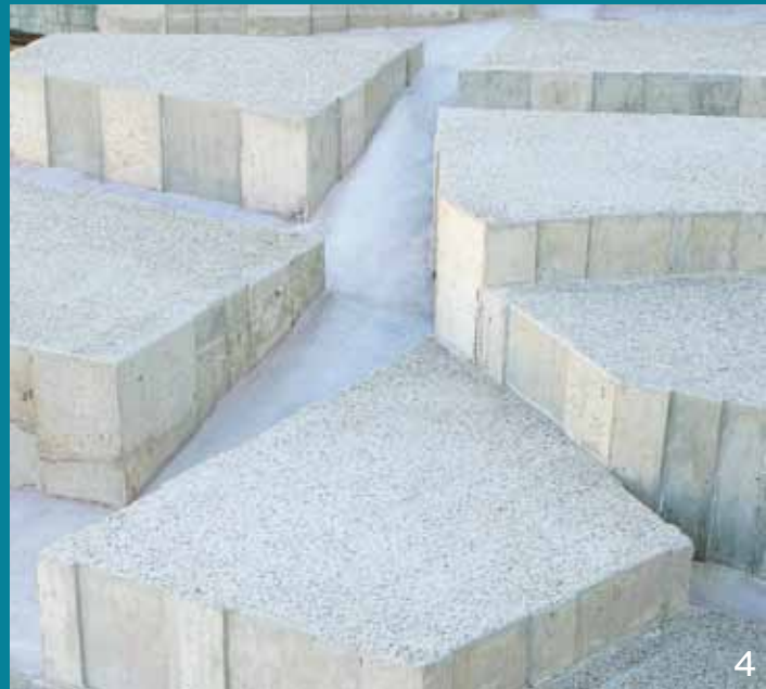
4 A stepping stone water feature has been created using coloured pre-cast panels (using CCS Parchment). Project: Ephraim Island. Landscape Architect: EDAW Australia.
