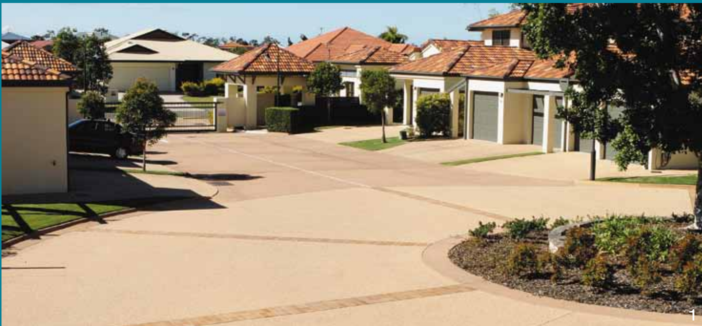
1 A combination of coloured exposed concrete and coloured concrete in a broom finish complements this townhouse development. Colour: CCS Biscuit.
