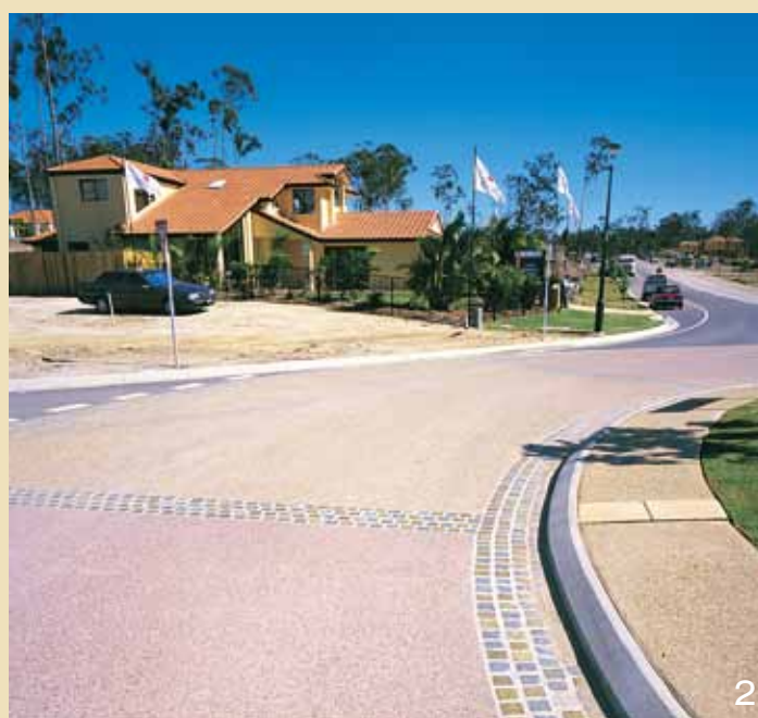
2 Natural granite cobble inserts were used in combination with dual coloured concrete to create a hard wearing but stylish roundabout entrance to this housing estate. CCS Biscuit and CCS Heritage Red were used to colour the concrete.
