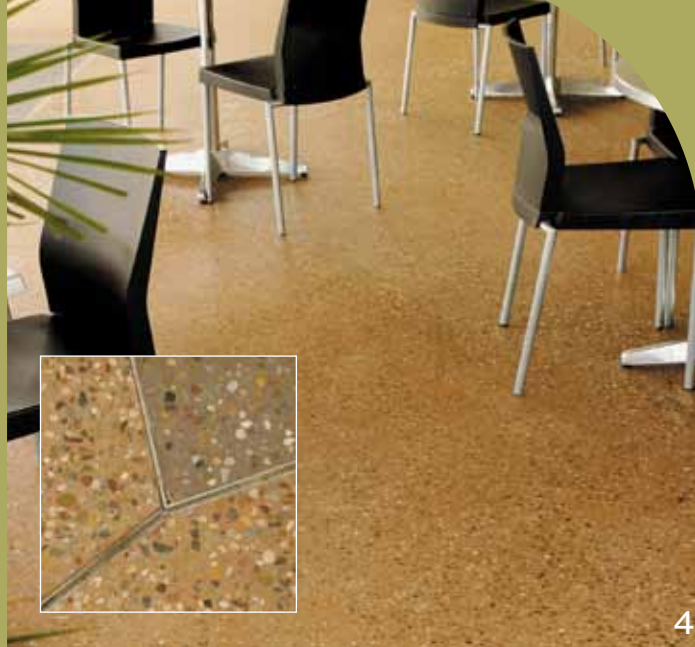
4 This cafe floor was first coloured, (CCS Biscuit and CCS Earth Brown) placed and then subsequently ground and polished to expose the natural aggregates in a smooth finish.
