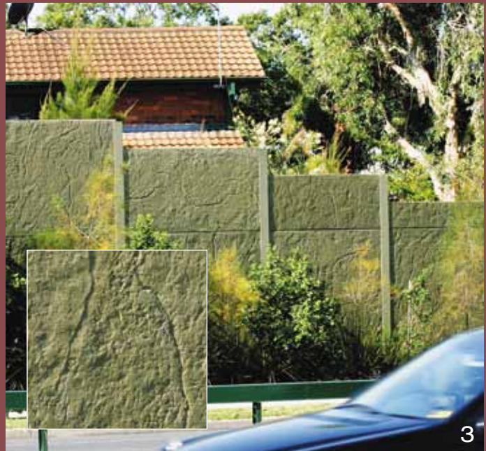
3 Combine function with form. Sound barrier walls at a busy intersection were coloured with CCS Eucalyptus and then textured with a CCS mega stamping mat. Subsequent plantings will grow with time to blend with the panels to create a unified, unobtrusive but functional sound barrier.
