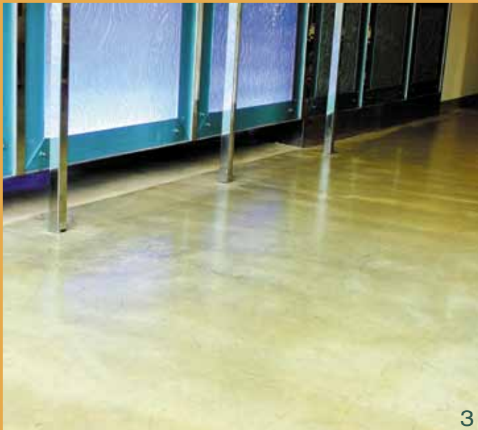
3 This contemporary bar room floor was created by first colouring it with CCS Custard, machine trowelling the surface and then sealing it with CCS Armourseal.
