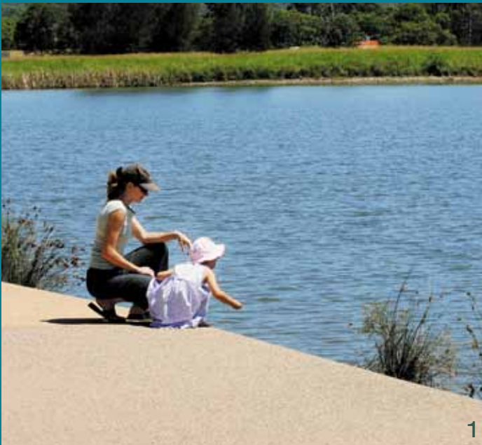
1 Coloured pathways add to the quality of family excursions. CCS Caramel and a predominantly white stone were used to create a coloured exposed finish.
