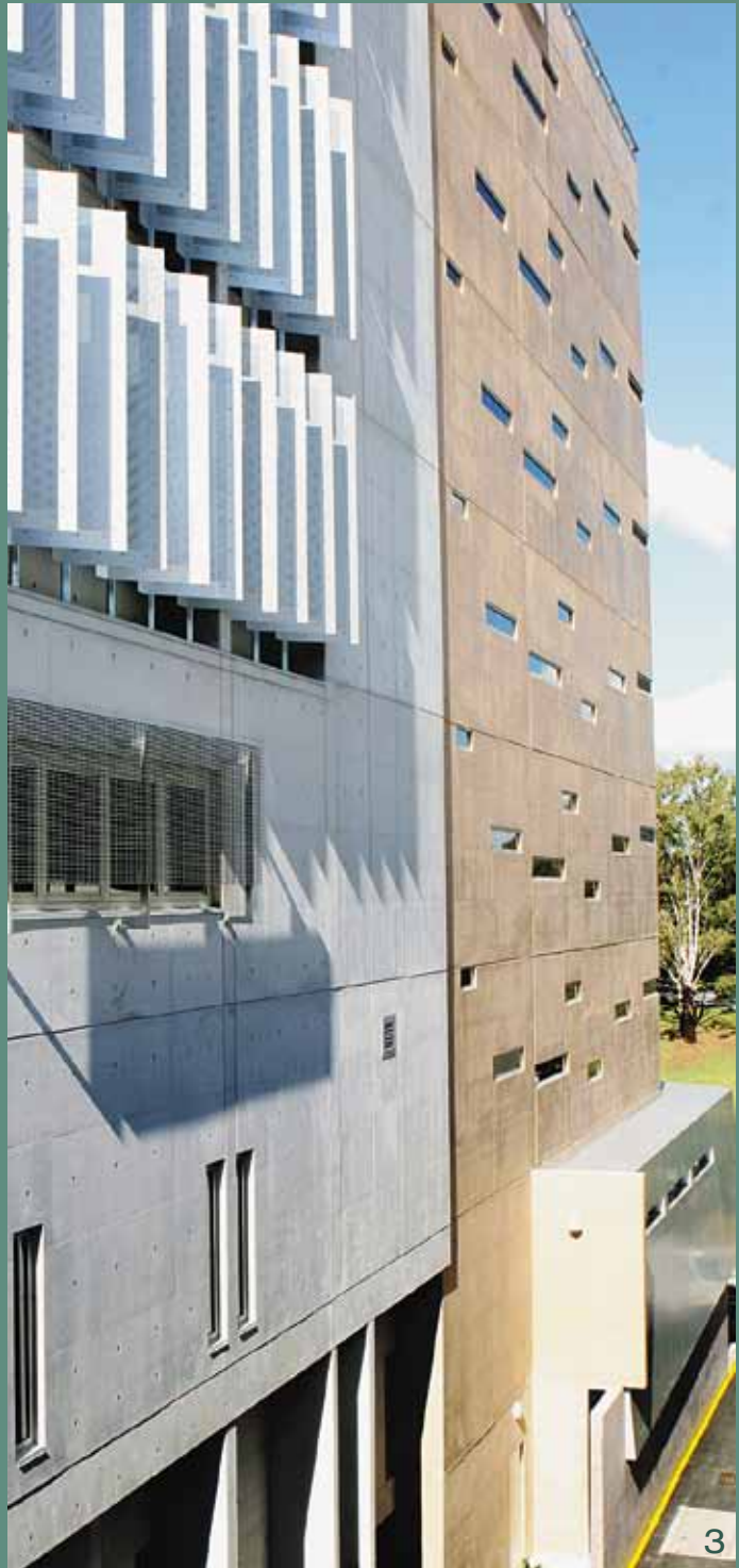
3 Special CCS colour blends were developed in conjunction with the project architects to create a facade that blends well with surrounding infrastructure. Project: James Foot Building, University of Queensland. Architect: Wilson Architects.
