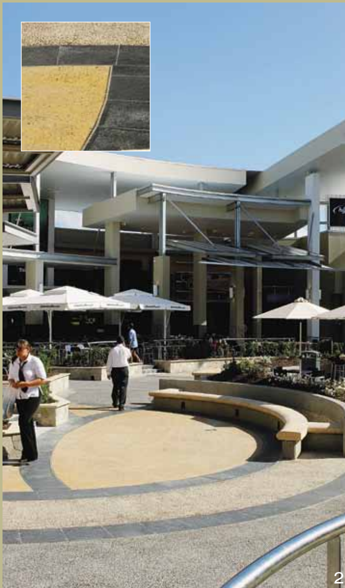
2 Garden beds and permanent seating were designed in conjunction with the coloured concrete floor to create an inviting exterior food court area. CCS Ghost Gum, CCS Onyx 21 and CCS Banana with off white cement, were used in conjunction with an exposed aggregate finish and charcoal coloured tiles. Architect: The Buchan Group.
