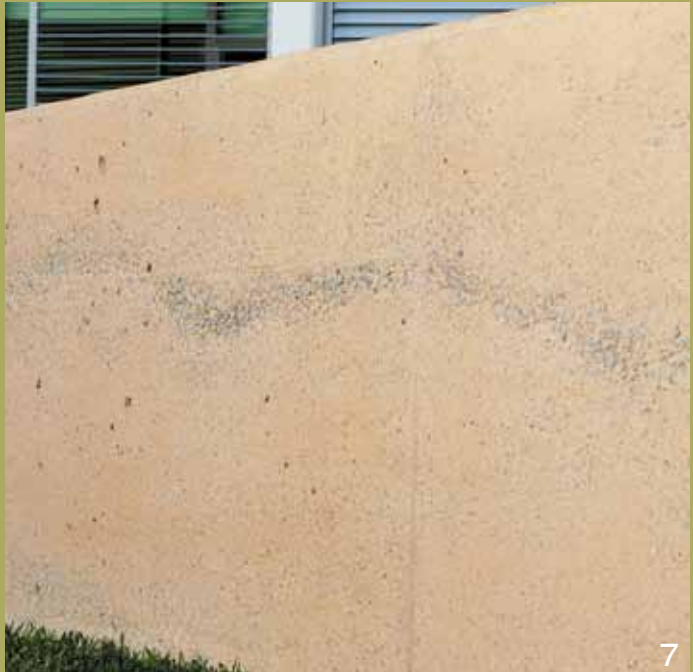
7 This feature wall has been coloured with CCS Biscuit and sandblasted for a textured effect. Architect: Edaw Australia.
