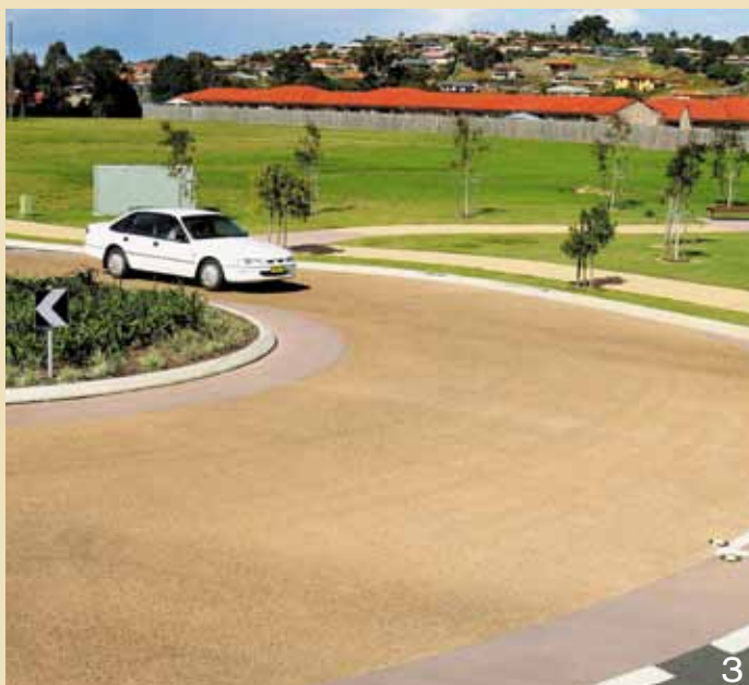
3 Roundabouts become feature areas that add character to estates when coloured concrete is used. CCS Biscuit and CCS Mulberry were utilised.
