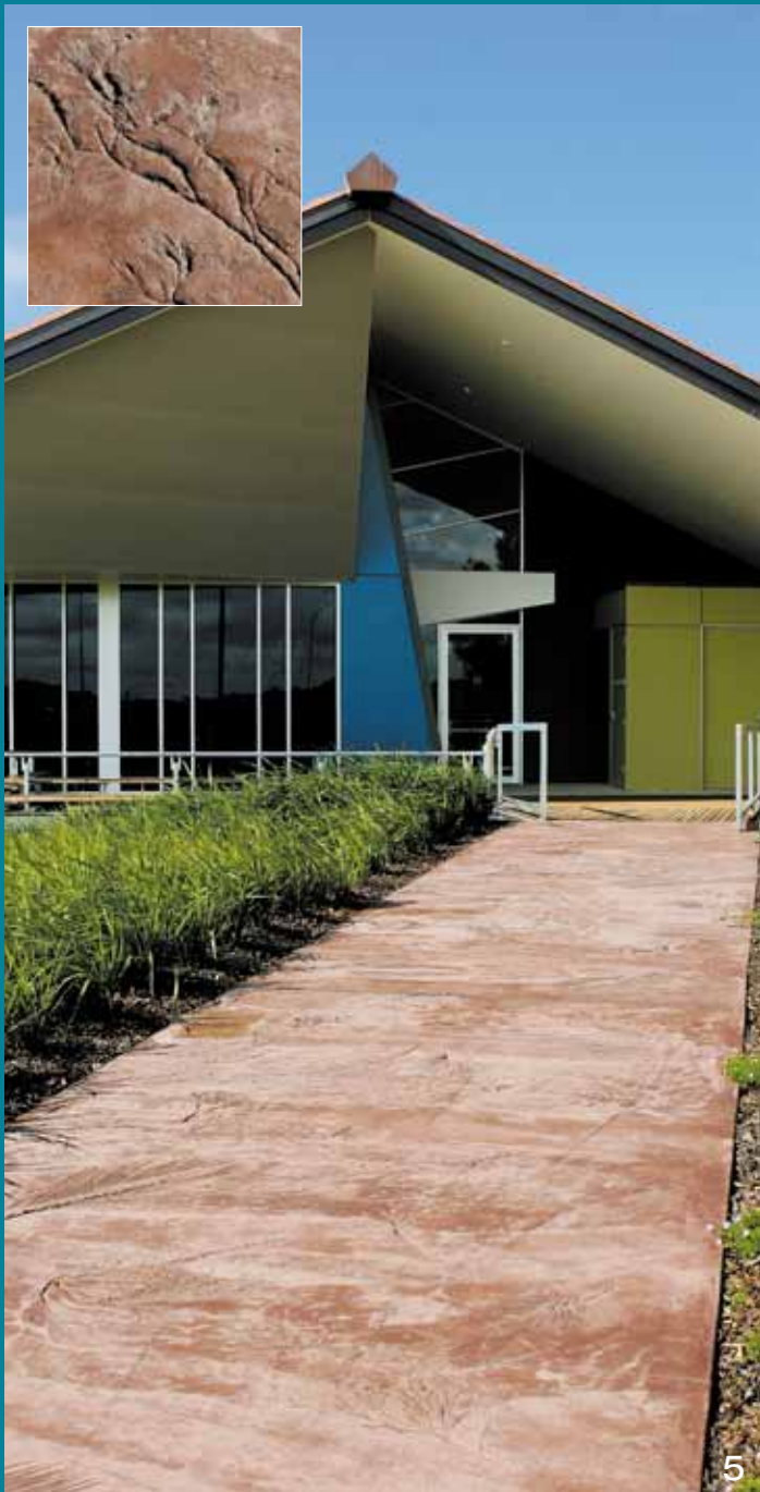
5 Local plant varieties were pressed into the wet coloured concrete and then removed to create a permanent natural surface impression. Concrete coloured with CCS Sandplain.
