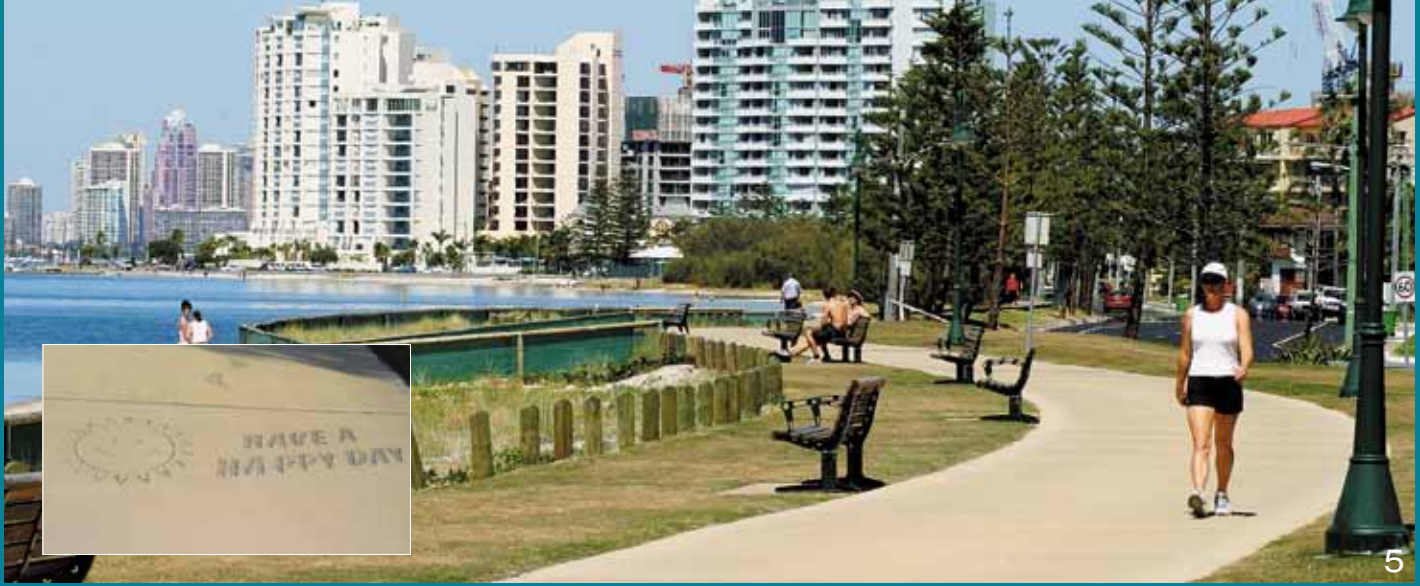
5 A template with a friendly greeting was placed on the dry coloured concrete and then sandblasted to permanently etch the message into the surface. CCS Desert Buff was used to colour the pathway.
