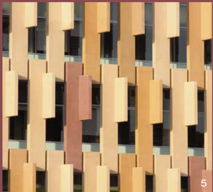
5 Colour combinations reminiscent of natural sandstone yet in bold geometric form were used to create these exterior panels. A combination of several CCS pigment blends were created in conjunction with project architects and cast off site. (CCS Mountain Rose, CCS Worstead Tan, CCS Mushroom Cap and CCS Silvery Moonlight) Architects: Donovan Hill and Peddle Thorp Architects.
