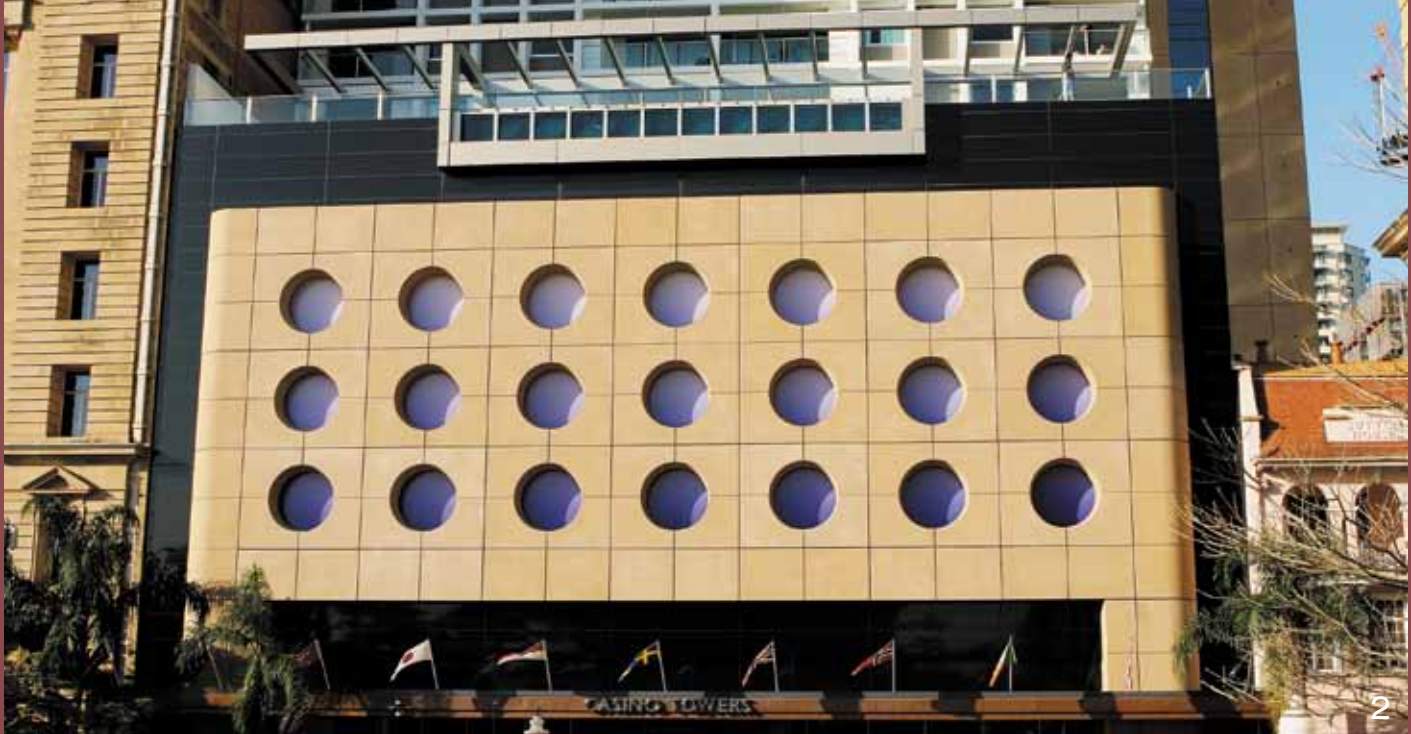
2 A wonderful example of how a simple but highly effective pre-cast panel design adds character to a building facade. Pre-cast panels coloured with CCS Honeycomb.
