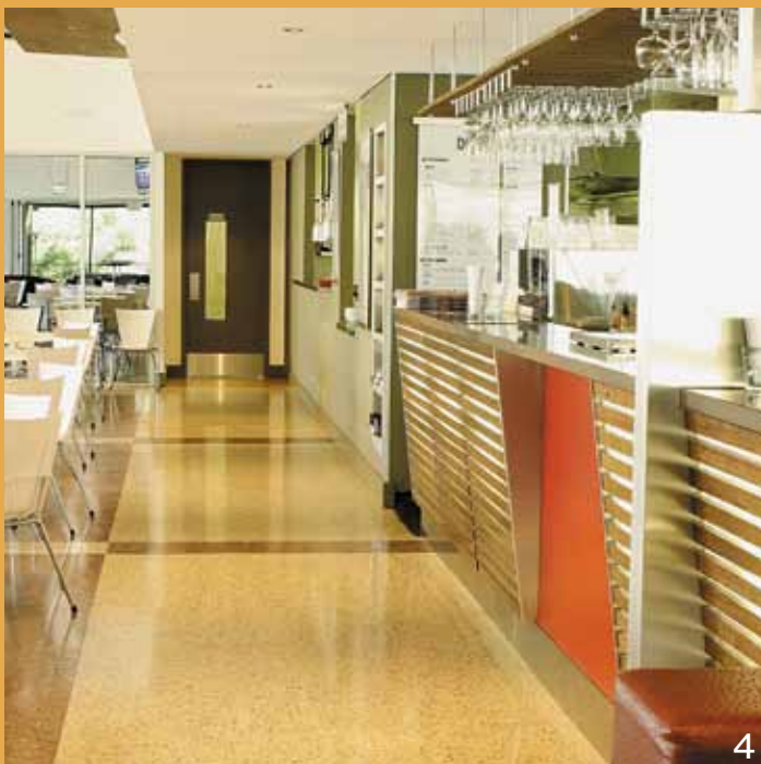
4 A combination of CCS Colours, special stones and placement technique resulted in a series of contrasting coloured floor panels. All were subsequently machine polished and then sealed.
