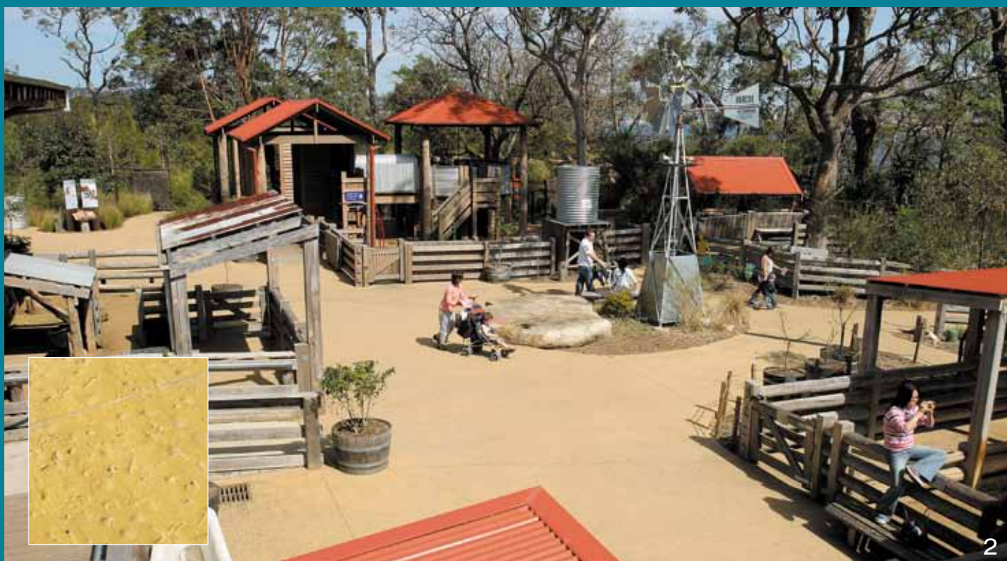
2 Another mega mat textured job – this time a 'salt rock' finish was used at Sydney's Taronga Park Zoo. CCS Morocco was used to colour the concrete.
