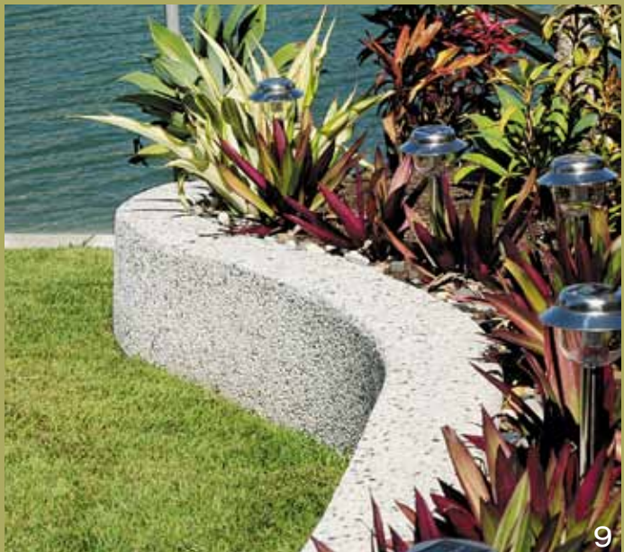
9 Integrally coloured garden walls were created on site coloured with CCS Pewter. The concrete surface was subsequently treated to expose the predominant aggregate.
