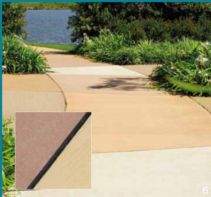
6 The character and appeal of this lakeside walkway has been enhanced through the use of multiple colours, CCS Caramel, CCS Honeycomb, CCS Desert Buff, CCS Pewter and CCS Earth Brown.
