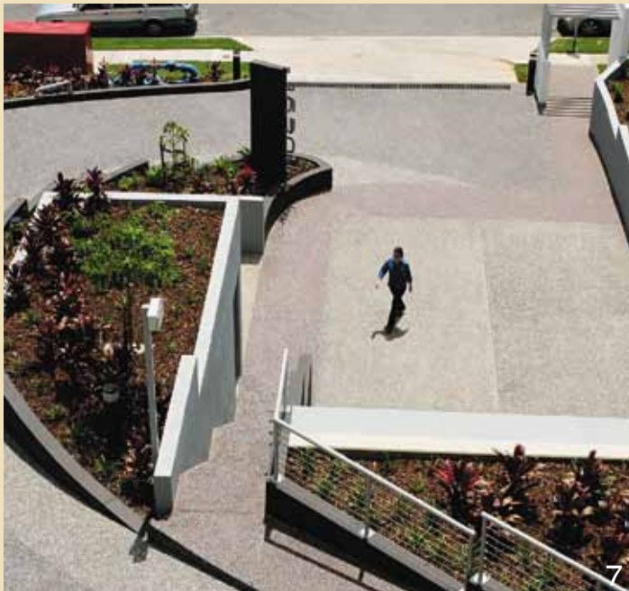
7 A great example of how several pours of different coloured concrete can be used in the one area. Natural stones and aggregate were exposed to add further colour and traction. Colours: CCS Grape, CCS Panther, CCS Pewter. Architect: Kevin Hayes Architects.
