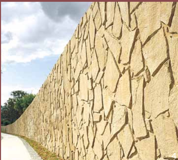
4 Patterns and textures were embedded into the concrete at the pre-cast concrete plant using specially designed forms and then erected on site. Colour: CCS Honeycomb.
