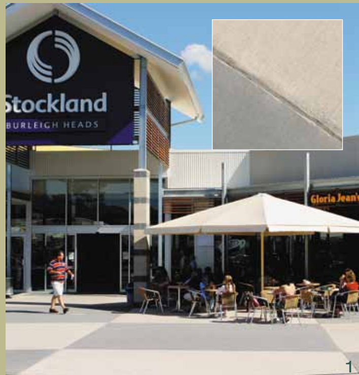
1 A large scale checker board pattern was utilised for this busy entry area. CCS Alpine and CCS Black 21 were used to colour the concrete.
