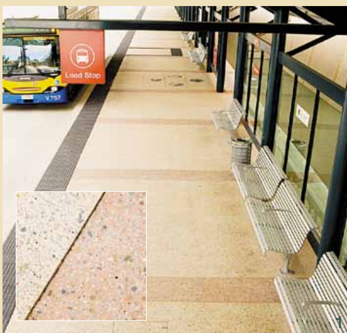
1 Coloured concrete was subsequently honed to produce a smooth and easily trafficable pedestrian area at this busy bus station. CCS Caramel and CCS Light Peach were the colours utilised. Architect: Peddle Thorp and Cottee Parker Architects. Landscape Architect: Tract Consultants.
