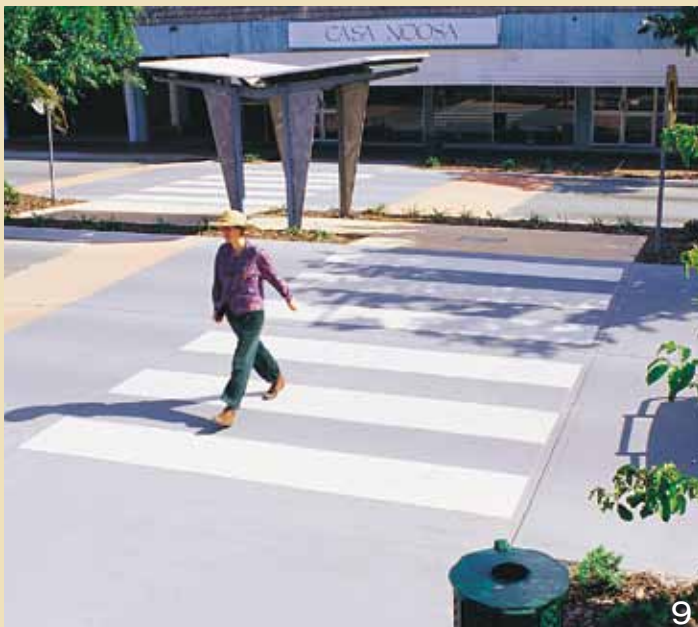
9 Elevated pedestrian crossings can be both functional and attractive when coloured concrete is used. Colours: CCS Black 21 for the crossing and CCS Pottery for the ramp.
