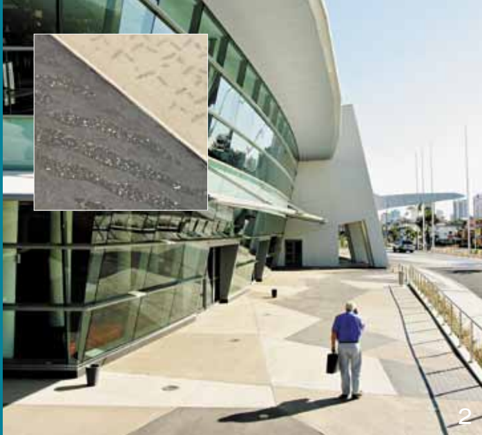
2 Local Gold Coast artist Mal Lecke was consulted by project developers to recommend colours and themes that were representative of the local area. CCS Lychee and CCS Panther were ultimately used and the concrete was subsequently sandblasted to reveal the white stone.
