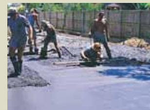
4 Coloured concrete is screeded and floated.
