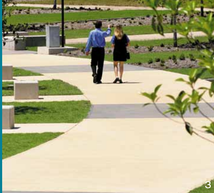
3 Bold contrasts in colour using CCS Lemon Cream and CCS Black 21 create a contemporary walkway through this regional park. Project: Seventeen Mile Rocks Riverside Park, Brisbane. Design Team: Brisbane City Council City Design Group.
