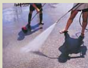
5 Where the "exposed aggregate" finish is desired, the surface layer is removed with water pressure.
