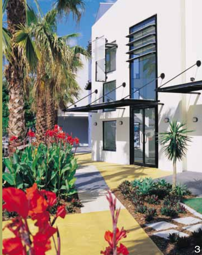
3 Coloured concrete was laid in a staged manner to create contrasting colours in a small area. CCS Corn, CCS Pewter and CCS Bluestone. Project: James Street, New Farm. Architect: Cottee Parker Architects, Brisbane.
