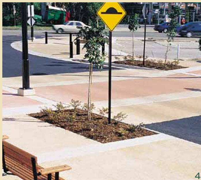
4 CCS Biscuit and CCS Brick Red were used in the footpath area, median strip and roadways to encourage and direct pedestrian and vehicular traffic flow.
