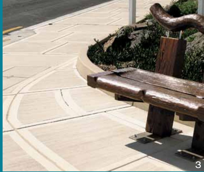
3 Secondary hand trowelling of the joints provides a coloured and textured contrast on this pathway. CCS Driftwood was used to colour the concrete.
