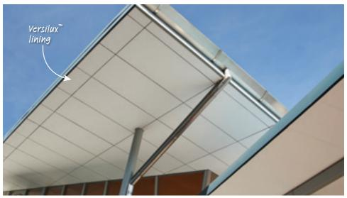
6mm Versilux<sup>™</sup> lining with James Hardie<sup>™</sup> Black PVC Eave and Soffit Jointer for an express joint look.
