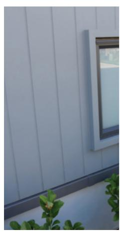
HardieEdge<sup>™</sup> trim is suitable for use in residential and selected commercial applications where compatible James Hardie<sup>™</sup> and Scyon<sup>™</sup> weatherboard, cladding and facade systems<sup>\*</sup> are fixed to a seasoned timber or light-gauge steel frame.
