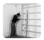
**3.** Fit the notches of the Clip profile (every 400mm).
