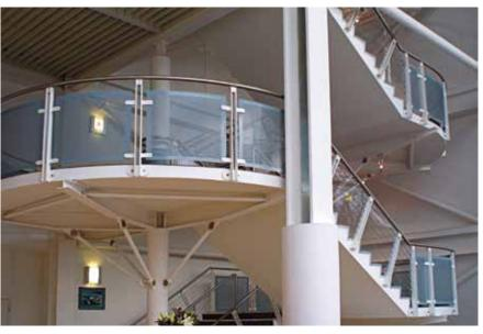
Balustrade infill panels with unperforated margins
